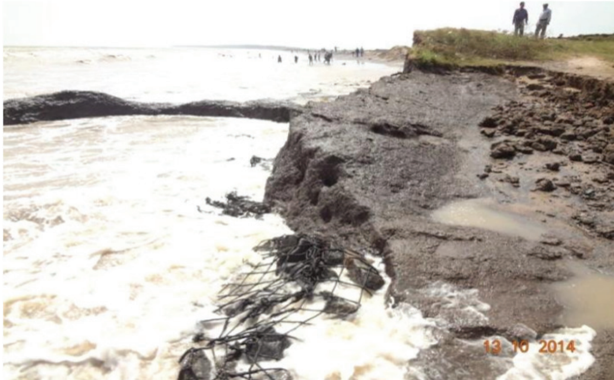
Figure 72 (b) Breaching of shoreline embankment on southern side of Pentha during Cyclone Hud Hud, on 12 October 2014 (Source: DoWR, Odisha)
