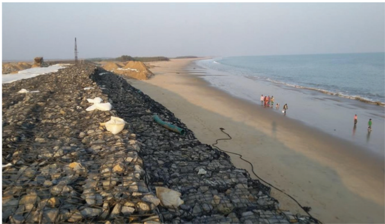
Figure 78 Accretion of sand has started in front of the geo-tube (Source: Department of Water Resources, Odisha)
