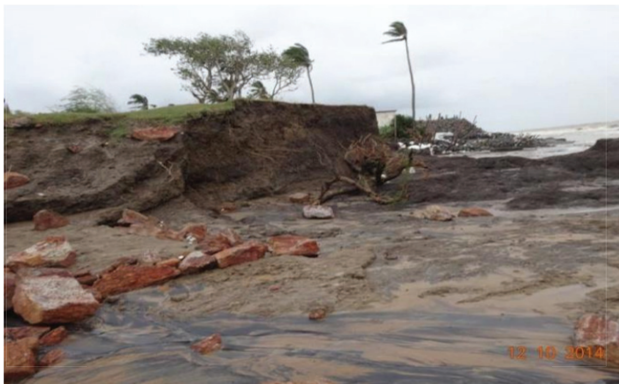
Figure 72 (a) Breaching of shoreline embankment on southern side of Pentha during Cyclone Hud Hud, on 12 October 2014 (Source: DoWR, Odisha)
