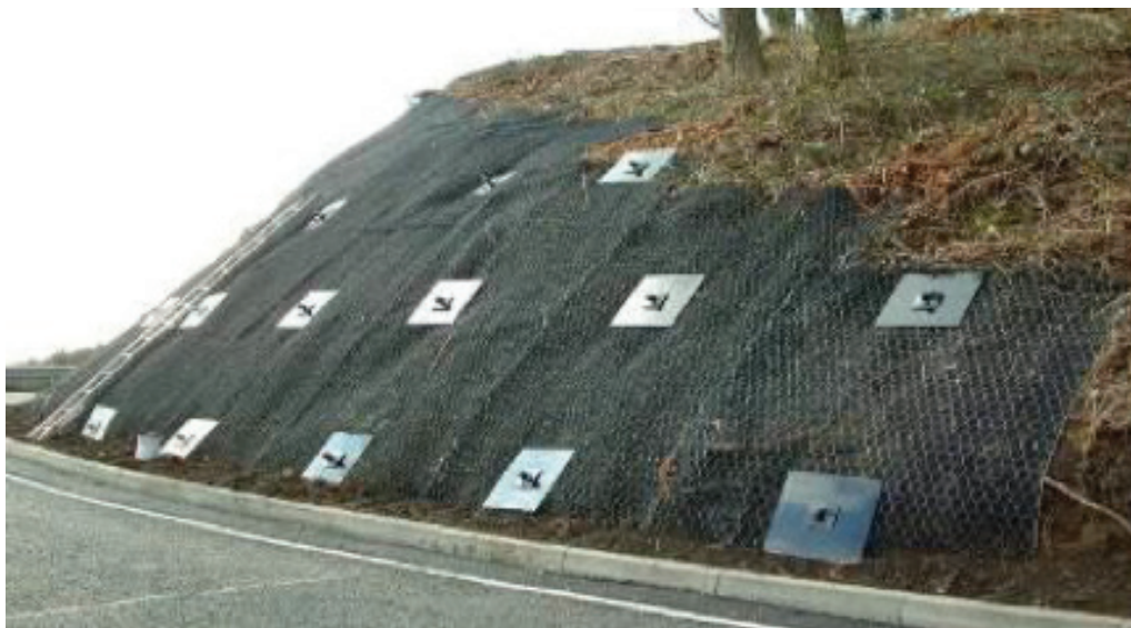
Figure 44 GI mesh anchored on the ground.
