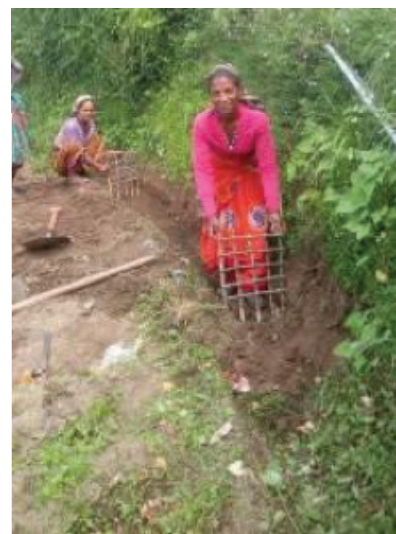
Figure 43 A view of toe trench work in Nainital District
